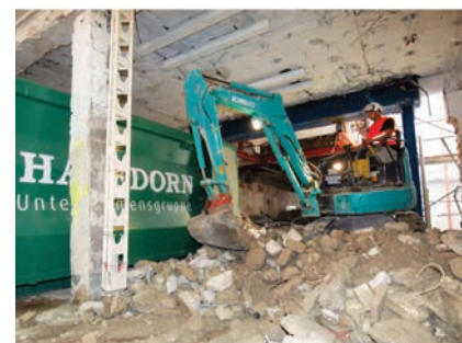
Germany's Hagedorn goes indoors at a job site in Dusseldorf
